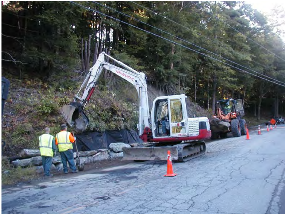
Rock retaining wall construction Brook Road
