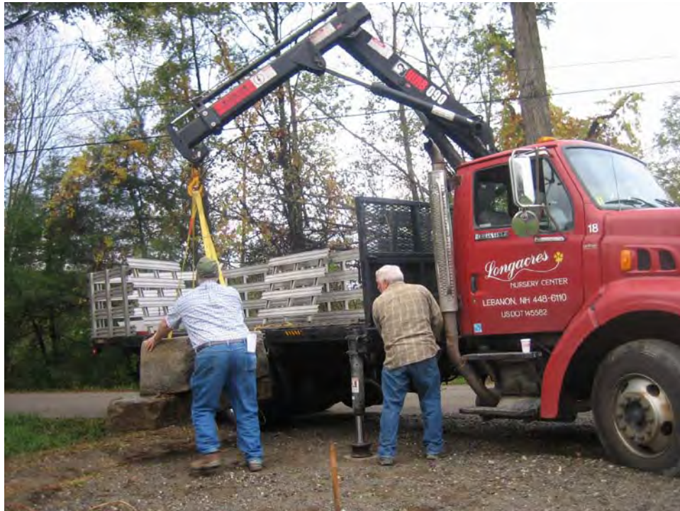
Granite watering trough being returned to Old County Road, Norm Longacre and Guy Daniels setting the stone. Photo S. Halleran
